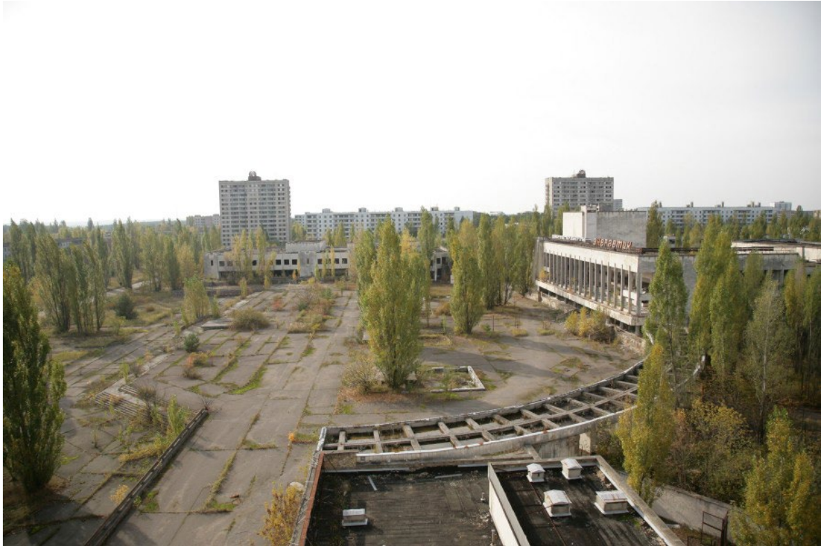
Figure 10. Image from Aesthetics Wiki entry “Soft Apocalypse”, which features as key motifs “overgrown cities” and key values “Hope, harmony with nature, anarchy, Nature taking it back”. The photo shows vegetation growing through concrete in the city of Pripyat, Ukraine. The city was abandoned after the nuclear disaster in Chernobyl in 1986.
