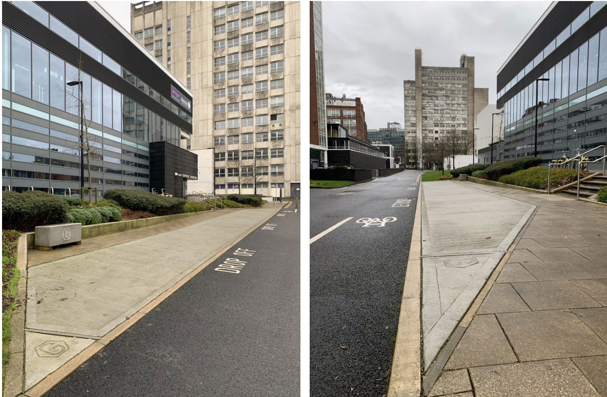
Figure 4 and 5 ‘Concretene’ parking bay outside the GEIC; photos taken by the author 31 December 2022
