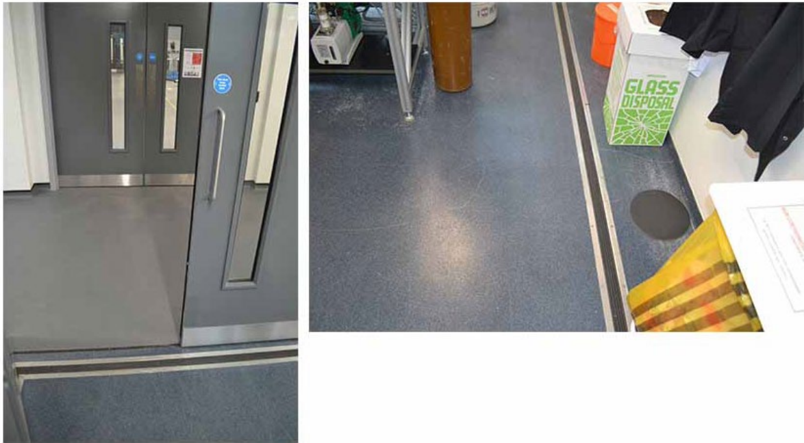
Figure 3: VC-D flooring around the perimeter of the Characterisation Laboratory; photos taken by the author, 21 January 2022
