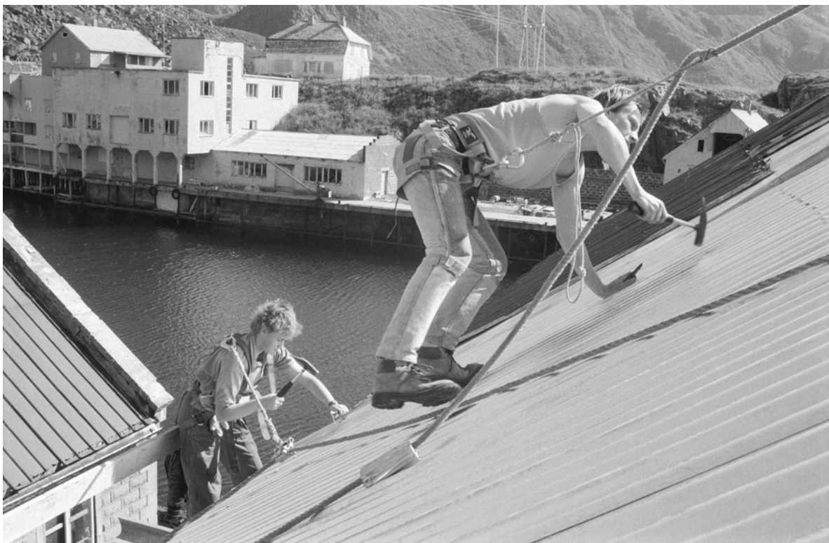
Photo taken by Wolfgang Eschenhorn, Roofing Work, 1987.
