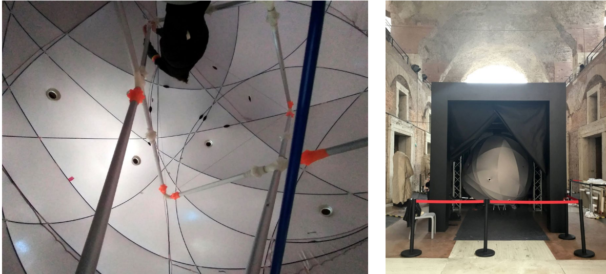
Fig. 4 and 5. Inner and exterior views of Synesthesia 's structural elements, its deformed geometry, and the surface wrapper. Photos taken during the artwork installation at the Trajan's Market Museum of the Imperial Fora in Rome.
